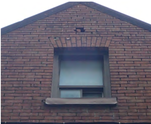
Fig.22: Metal covering over sill. Note bricks missing above segmental arch. West elevation.
