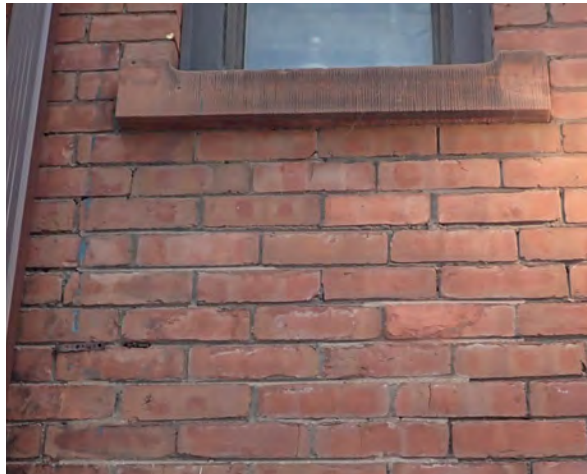
Fig.17: Bricks starting to spall. Note minor spalling to stone sill. West elevation.
