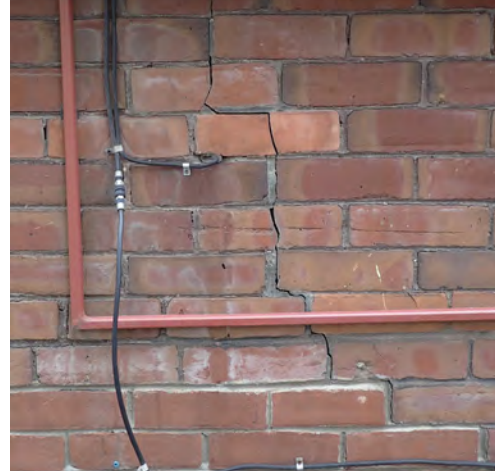
Fig.21: Example of crack in bricks between basement lintel and first floor sill. West elevation.
