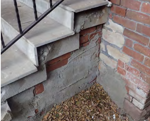
Fig.14: Unfinished side of steps. South elevation.
