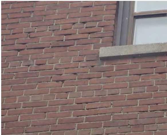
Fig.28: Open mortar joints. North elevation.
