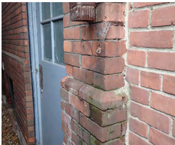
Fig.30: Missing down pipe connection. Note saturated masonry, and open mortar joints. East elevation.
