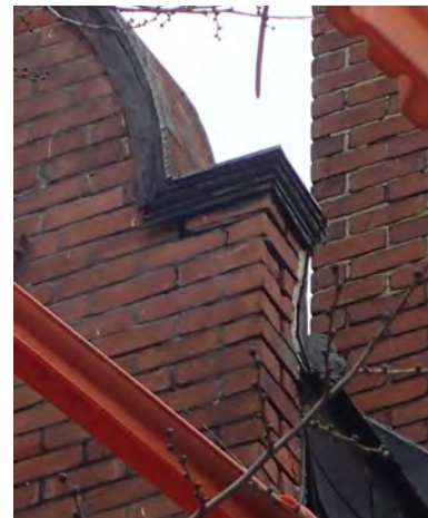
Fig.3: Open mortar joints at edge of Dutch gable. Note rusting flashing.
