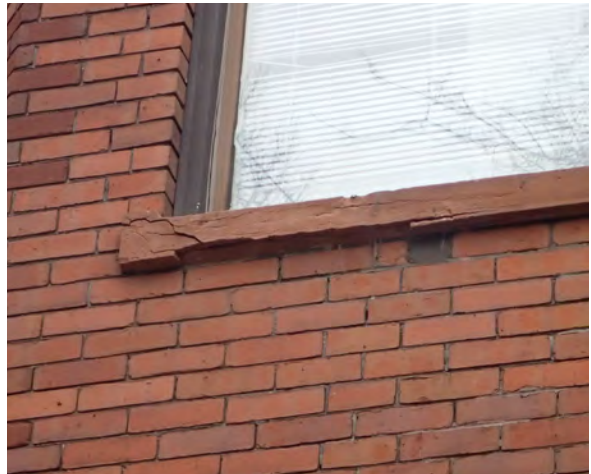
Fig.11: Spalled and cracked stone sill. South elevation.
