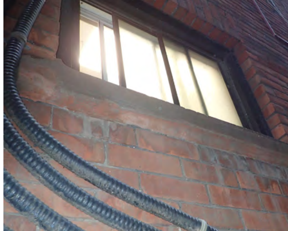
Fig.33: Defective stone sill missing base. East elevation.
