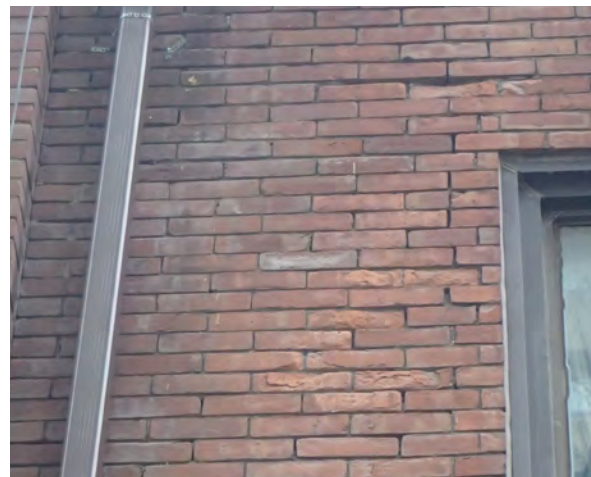
Fig.23: Example of spalled bricks. West elevation.
