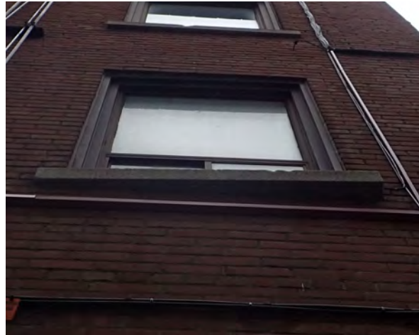
Fig.27: Example of sill out of alignment. West elevation.
