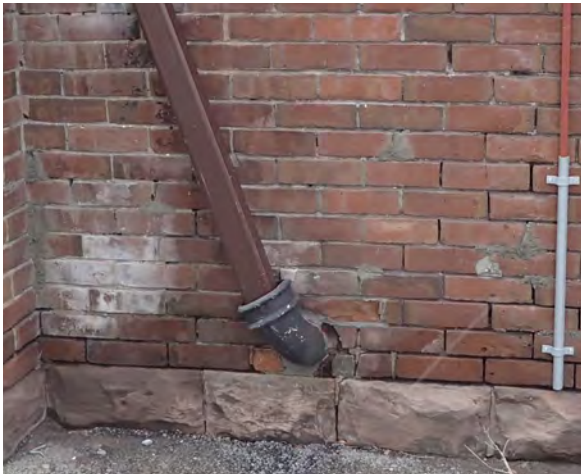
Fig.16: Open mortar joints in brick and stone, spalled bricks, and stained bricks. West elevation.
