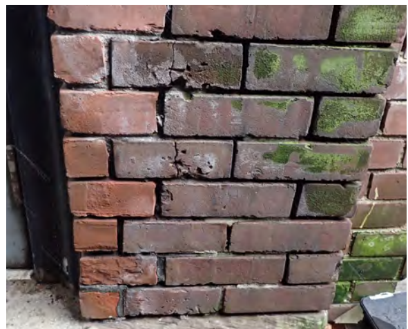
Fig.31: Vegetation staining to bricks, open mortar joints, and spalled bricks underneath down pipe. East elevation.
