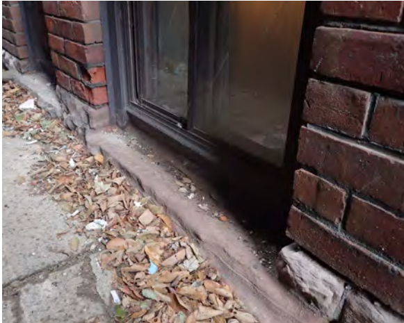
Fig.32: Spalled and defective stone sill, and spalled bricks. East elevation.
