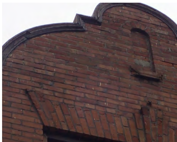
Fig.13: Fair condition of masonry at Dutch gable. Note over painted cornice.
