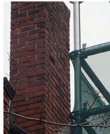
Fig.6: Open mortar joints in chimney
