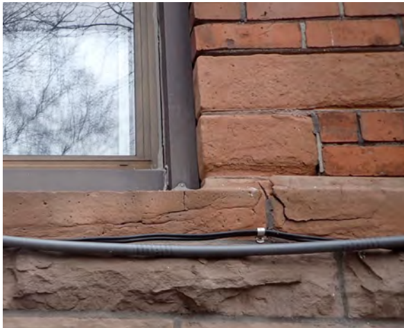
Fig.10: Spalled and cracked stone. South elevation.
