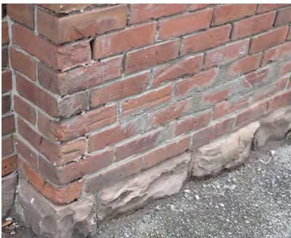
Fig.18: Spalled and damaged bricks at corner; open joints in mortar, and poorly repointed joints. West elevation.
