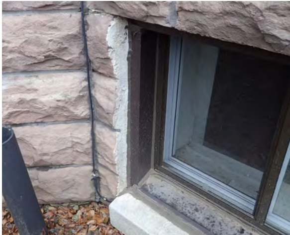
Fig.8: Parging to stone where cut for enlarged basement window. South elevation.
