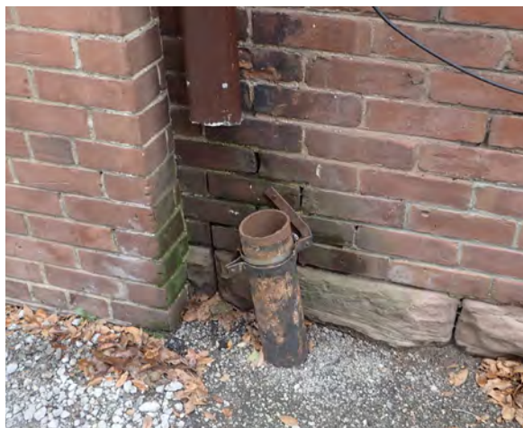
Fig.24: Missing downpipe connection. Note saturated masonry, and open mortar joints. West elevation.
