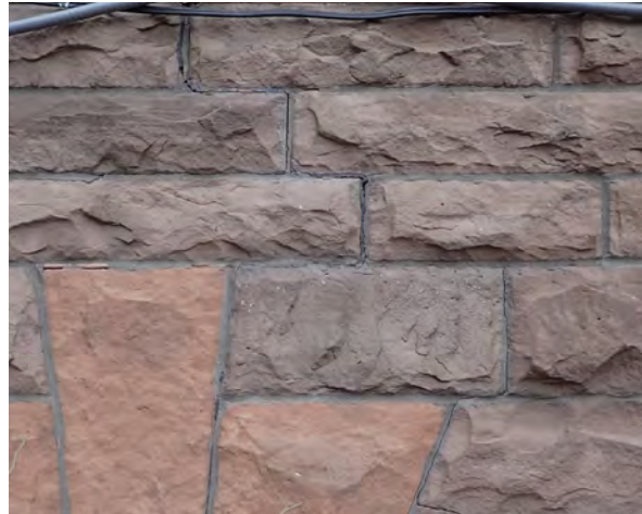
Fig.9: Stepped crack through mortar joints. South elevation.
