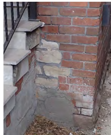
Fig.4: Open mortar joints, patch repair, and poorly matched replacement material for bricks.
