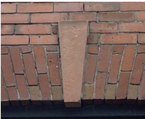
Fig.12: Minor surface deterioration to keystone. South elevation.
