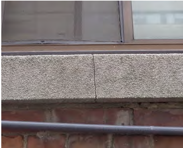
Fig.26: Example of cracked sill. West elevation.
