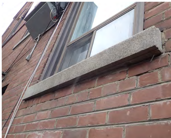
Fig.35: Concrete sill out of alignment. East elevation.
