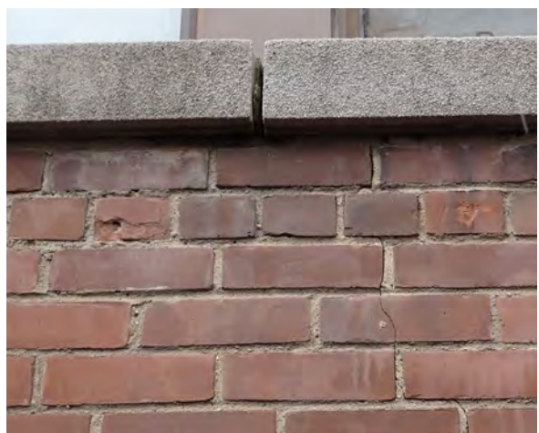
Fig.29: Hairline crack in bricks, and open mortar joint in sill. North elevation.
