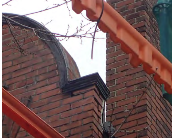
Fig.15: Rusting flashing to cornice. South elevation.
