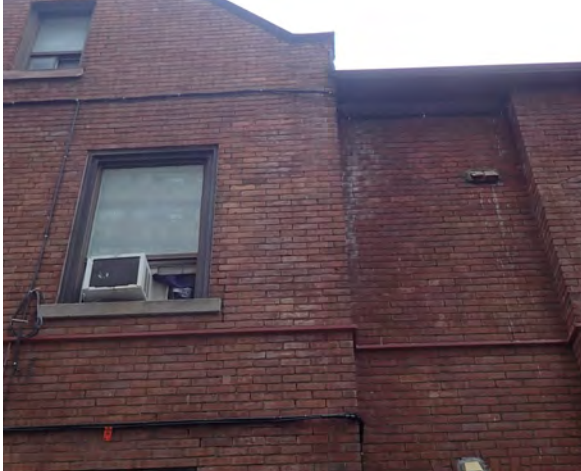
Fig.20: Staining to bricks. West elevation.
