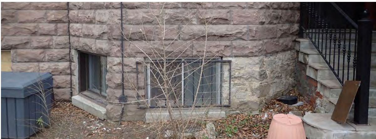
Fig.7: General condition of stone at basement level. Note poorly selected replacement material adjacent to steps. South elevation.
